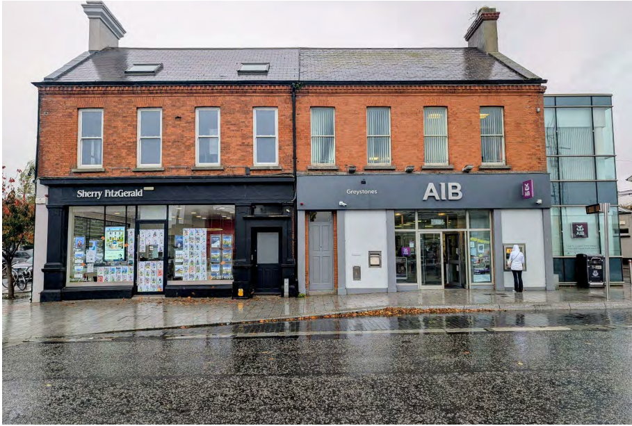
1. Traditional Shopfronts (Purpose-Built): As a former residential street, Church Road contains relatively few historic, purpose-built shopfronts. A notable example is the Victorian red-brick building that formerly housed McFarlands and Murphy's Newsagents, which stands out as a distinctive feature along the street. Such buildings should be prioritised for the reinstatement of traditional shopfronts to reinforce the historic character of Church Road.
