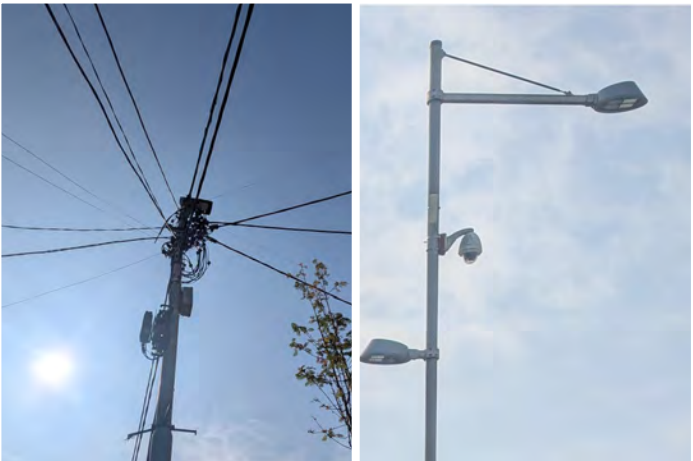
Image 4.7-4.8: Existing street lighting on Church Road. Lower Church Road (right) upper Church Road (left).
