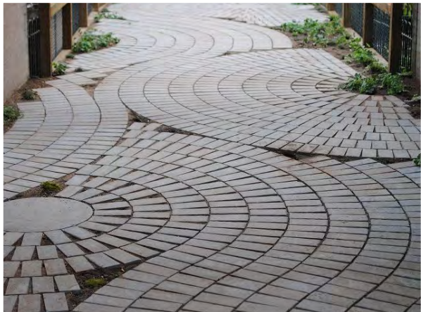
Images 6.9-6.10: Incorporating patterns into laying of granite setts in verge and spill-out areas, such as fan effect, can provide a subtle reference to the coastal location and act as a directional tool.
