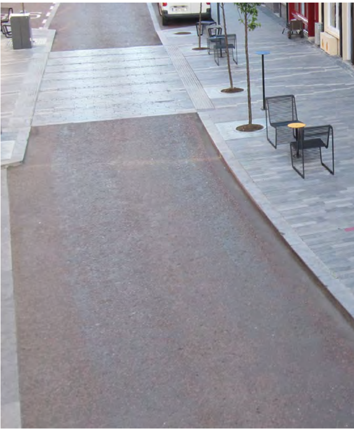
Image 1.1: Coloured asphalt defines inner town carriageways with courtesy crossings at regular intervals emphasising pedestrian priority (Clonakilty, Cork).
