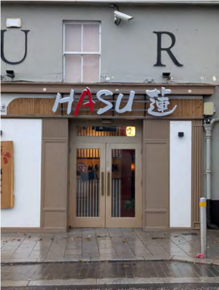
Image 8.3: Modern shopfront inserted into a historic building on Church Road, lacking coordination with the context and inappropriate within the historic setting.
