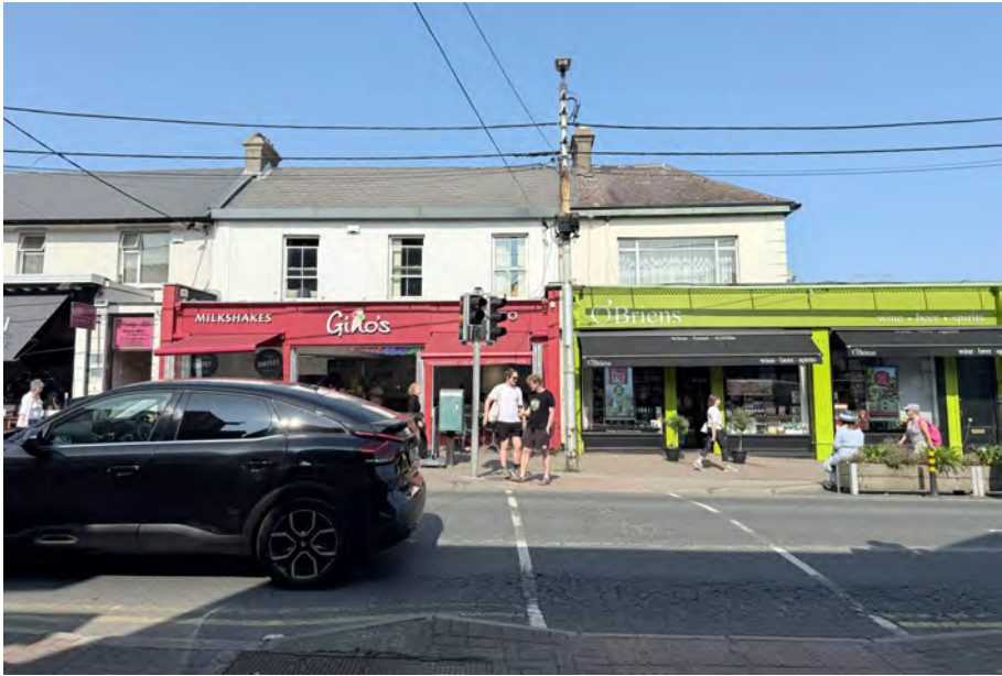
Former Residential Buildings (Shopfront Extension at Ground Floor): Many former residential properties along Church Road have been adapted with ground-floor shopfront extensions to accommodate commercial use. These interventions vary in quality and often disrupt the original façade composition, but they retain elements of the building's historic form above the shopfront. Where carefully designed, such extensions can provide active street frontage while maintaining the overall character and rhythm of the streetscape and relationship with upper levels.
