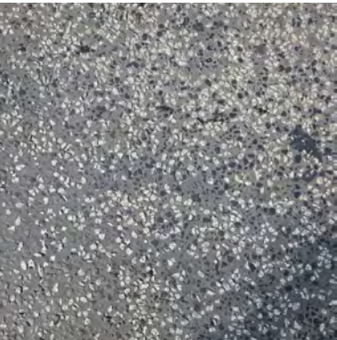
Carriageway Asphalt with aggregate chips
