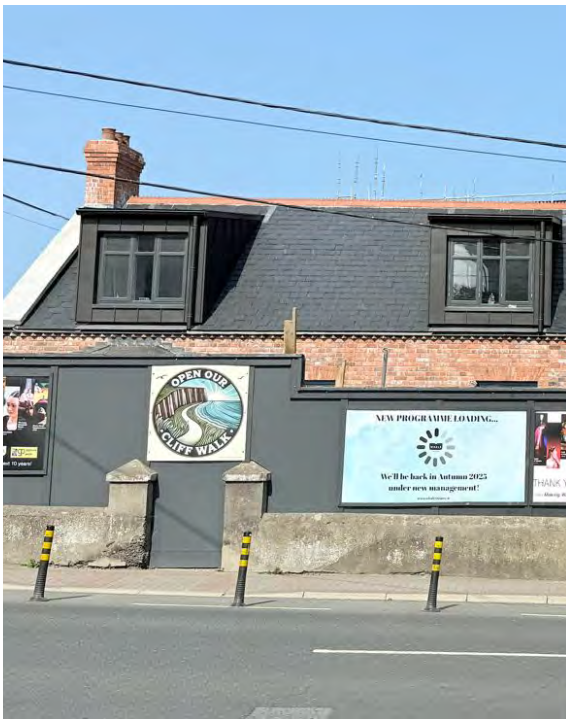
Helena Cottage (c.1880) - currently under construction
