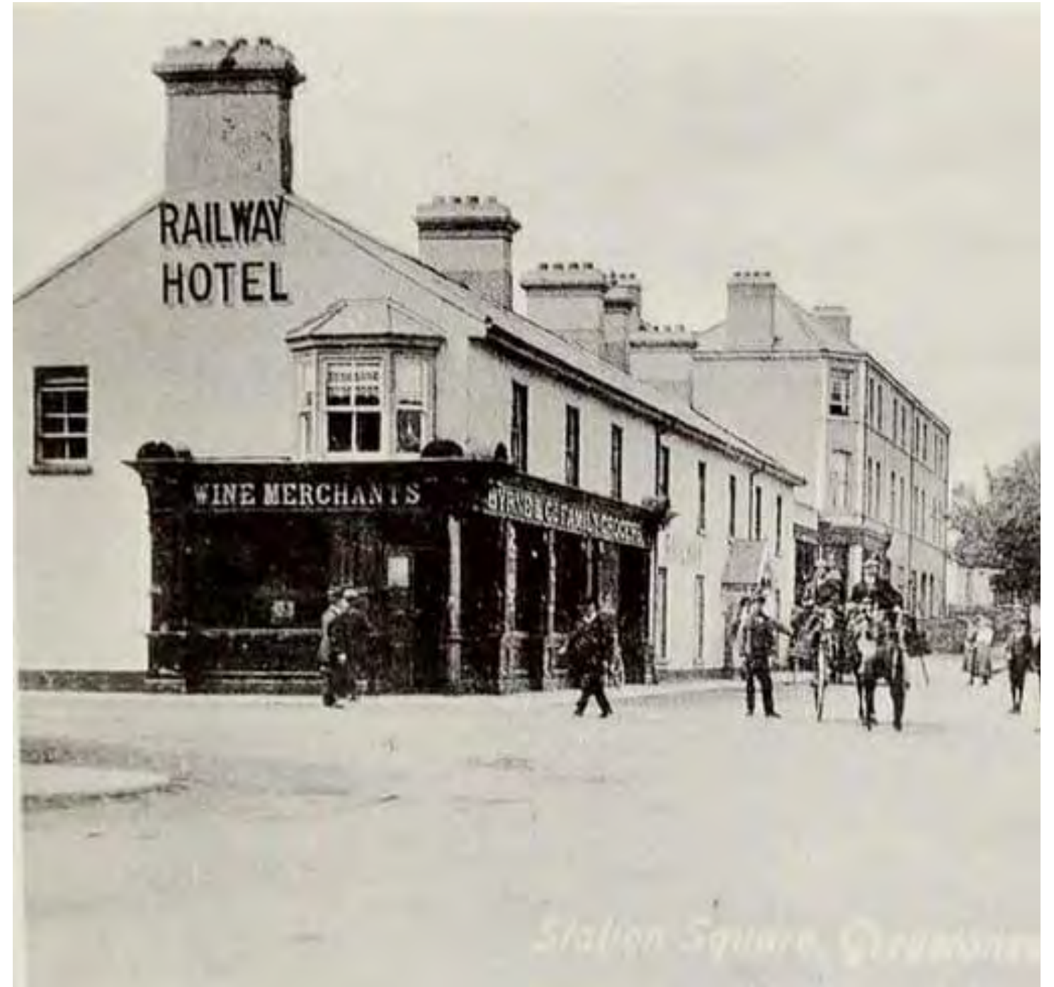
Station Square, historic shopfront
