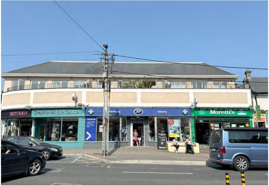
Modern Shopfronts (Purpose-Built): Purpose-built modern shopfronts along Church Road are generally larger in scale and use contemporary materials, often lacking the traditional proportions and detailing of historic shopfronts. While they contribute to the commercial function of the street, their design frequently contrasts with adjacent heritage buildings, affecting the cohesion and visual rhythm of the streetscape. Careful consideration of scale, materials, and façade articulation could help these buildings better integrate with the historic character of Church Road.
