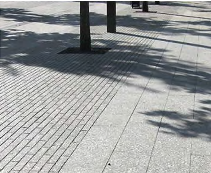
Image 2.2: Subtle approach to demarcation between footpath and verge zones through changing the scale of pavers.
