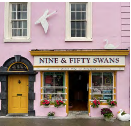
Image 8.5: Effective use of colour between shopfront lettering, features, and the overall building, complementing the architectural composition (Gort, Co. Galway).
